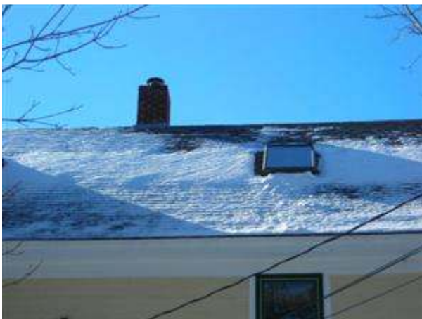
1.0 Picture 1 Limited visibility of roof due to snow covering.
