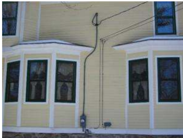
2.0 Picture 2 Side view of home showing the service entry.
