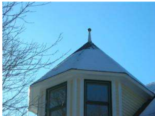
1.0 Picture 2 View of the roof.
