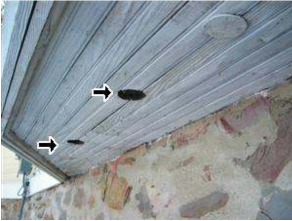
2.0 Picture 9 Missing insulation plugs should be repaired. 2.0 Picture 10 Minor dry rot observed under front porch.
