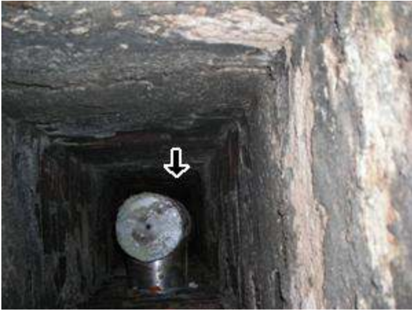
4.0 Picture 1 Interior view of the chimney/metal vent for furnace.
